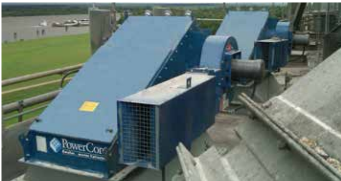
CPV-6 - Direct bin venting distributor head 2,400 cfm (4,077 m 3 /h)
