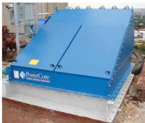
CPV-12 - Cement silo bin vent conveyor 3,700 cfm (6,285 m 3 /h)
