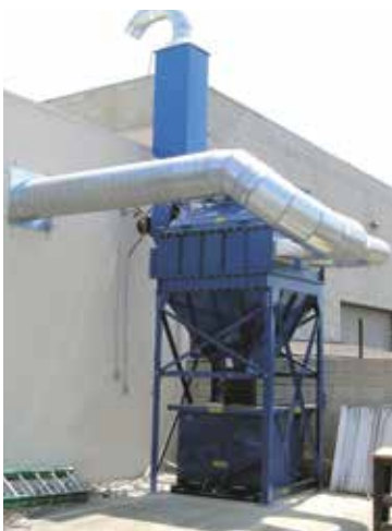
CPC-12 on Wood Dust at furniture manufacturer 7,000 cfm (11,891 m 3 /h)
