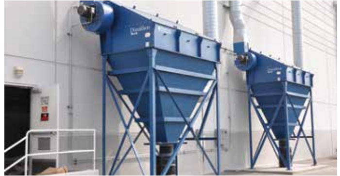
CPC-24 - Paper tissue manufacturing 7,600 cfm (12,910 m 3 /h)
